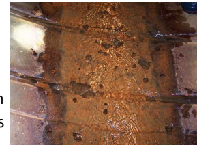
Figure 2.3-2 – Steel Pipe with Invert Perforations
