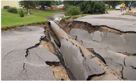
Figure 4.3-6 – Failure Due to Piping (Water flowing along outside of pipe and washing away backfill) (Photos courtesy of FEMA)
