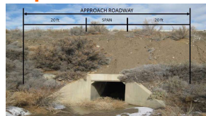
Figure 4.3-1 – Approach Roadway Inspection Length
